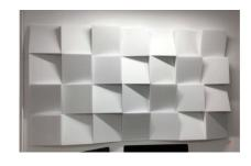
130 m<sup>2</sup> sound-absorbing panels with <u>equivalent acoustic parameters</u> as SKUM Acoustics Kilen, to be fixed to the wall and built as moving dividers or walls.
